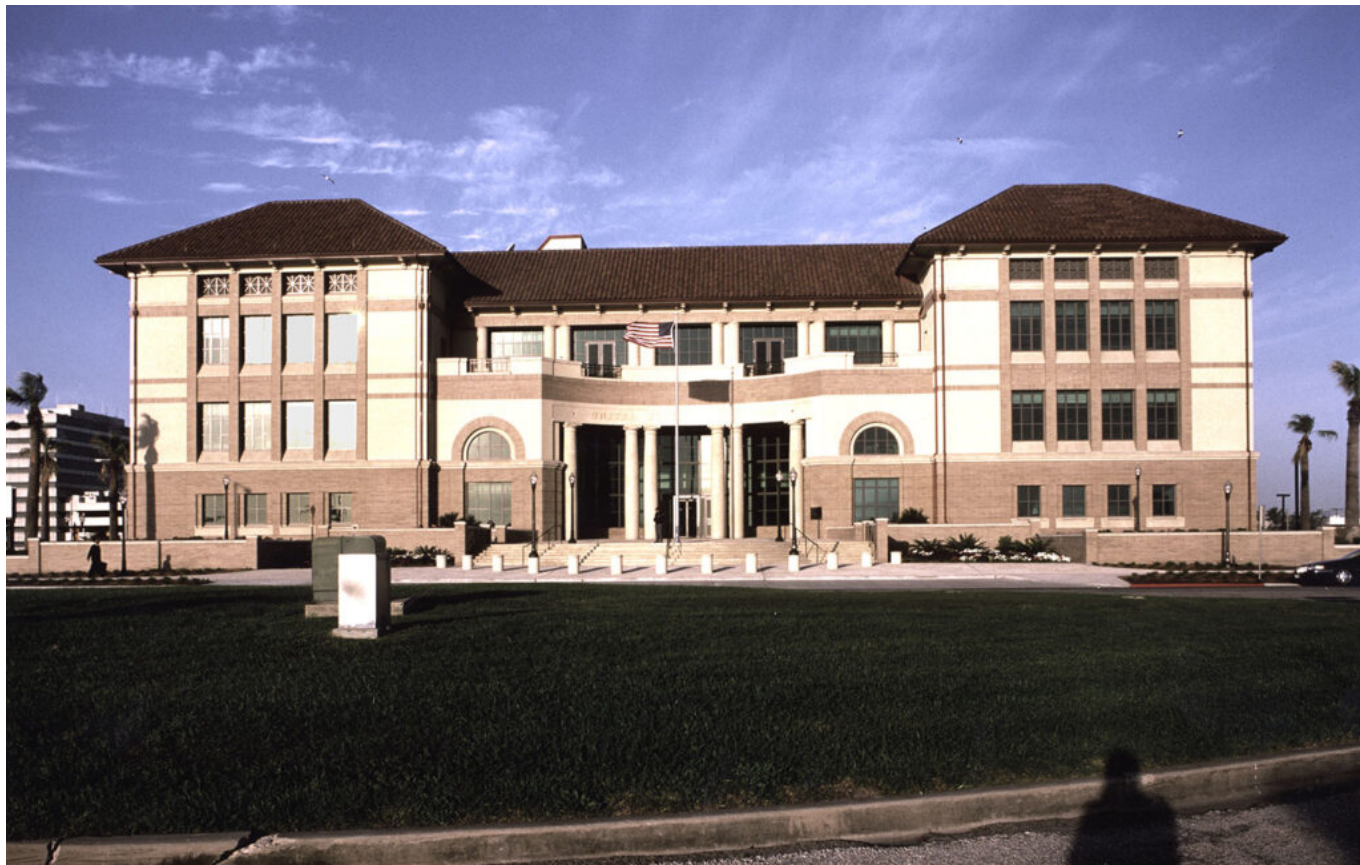
Hartman-Cox Architects, Corpus Christi Courthouse
